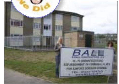
Pictured: Housing Services officers Kat Aylward and Philippa Dale outside the completed block and before and after shots.
