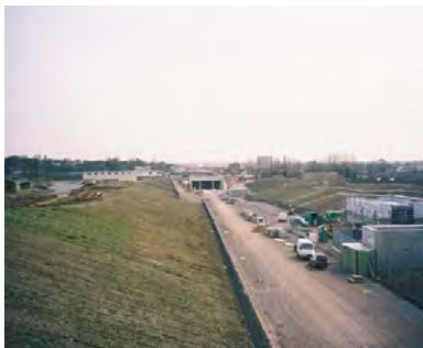
View along CTRL during construction
