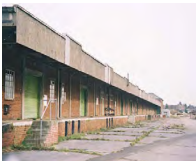
Existing Storage Sheds on former Rowcroft Barracks
