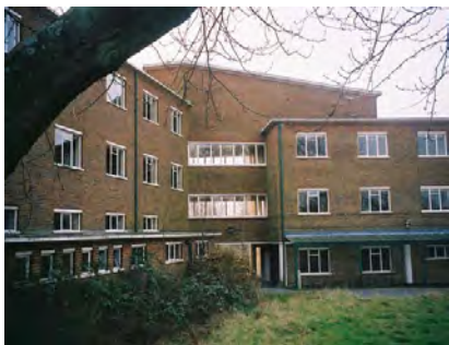
Existing accommodation block
