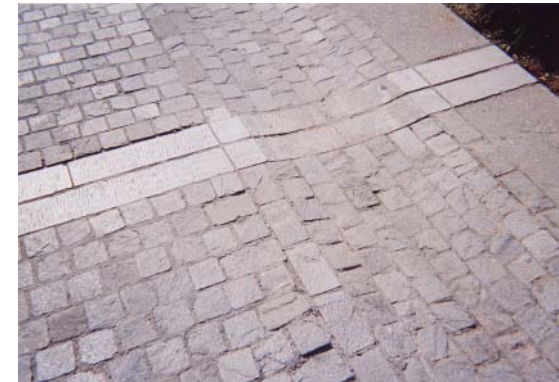
Flush surface to create integrated street surface
