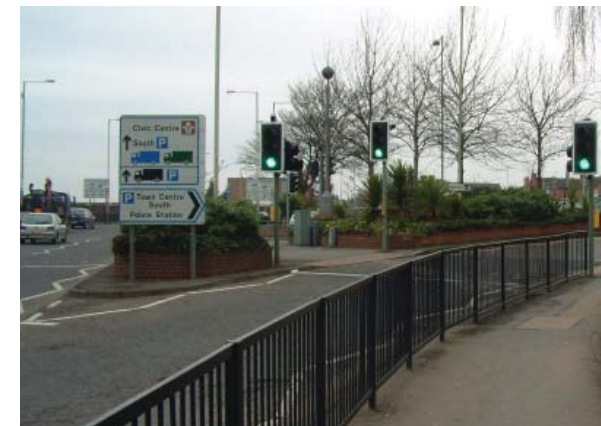
Visually dominant highway infrastructure
