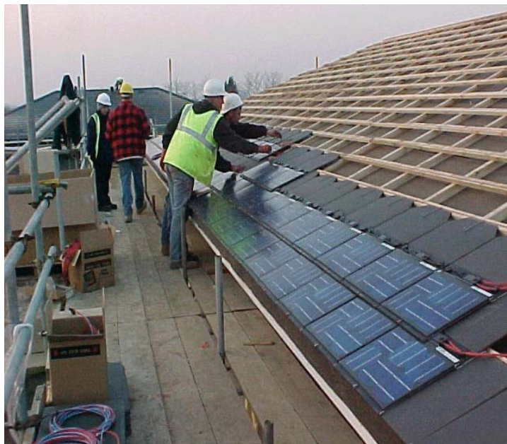
Installation of solar photovoltaic sunslates
