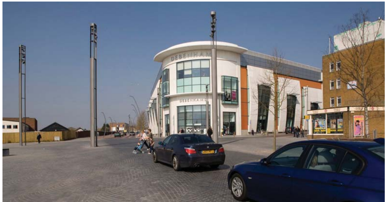
Elwick Square- Completed works
