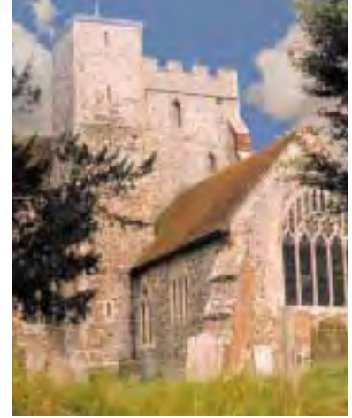
5. All Saints' Church, Boughton Aluph. First built in the 13th century of flint and rubble with ashlar dressings.
