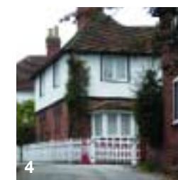
1 Brick porch 2 Doorway at Belke House 3 Doorway at the Talisman shop 4 Early nineteenth century Clements Cottage
