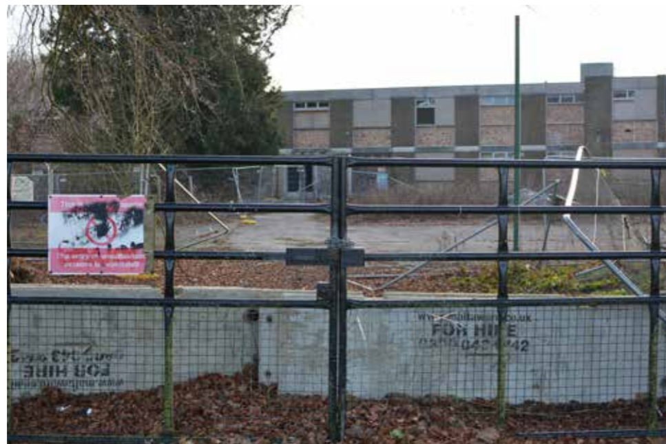
Photo 1: View east across the former ADAS site from Olantigh Road.
