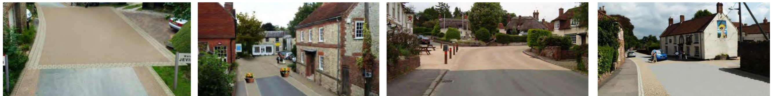
Slower streets and lanes – carriageway narrowing, contrasting materials, cross overs, pedestrian priority.
