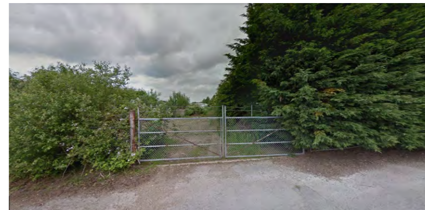
2 View looking through gate at existing obsolete research buildings
