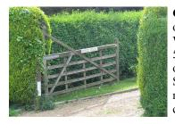
**Gates** - There are very few ornamental metal gates in Woodchurch. Most are simple 5-barred field gates made of oak or elm or soft wood painted. Some are picket gates set in a matching fence or in a low clipped hedge.
