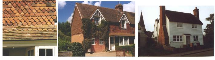
**Tiling** - The colours of most roofs blend with that of the walls. A number of houses have traditional hanging tiles on walls, either plain or elaborately patterned in a variety of shapes, replacing the decayed lath and plaster. This use of hanging tiles is usually confined to the upper floor. It improved weatherproofing for early timber-framed buildings and, by avoiding brick, reduced the total weight of the structure on unstable clay foundations.
