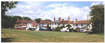
Most of these houses on the north-eastern side of the Green exhibit common building themes that can be found frequently in the Weald including Kent peg-tiled roofs, simple weatherboard-clad elevations and the use of timber framing.
