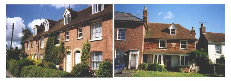
Early roof styles include the steep catslide (top left) and the popular half-hipping (some examples here on this page). Hipped and gable dormer windows make most of the roof space and are usually clad on the cheeks with rendering or hung tiles. Some late 19th-century houses have slate roofs. Locally few houses dominate their neighbours. There is sympathy between buildings in terms of scale. Few cottages exceed 4 metres in height at the eaves level and 6 metres at the roof ridge.
