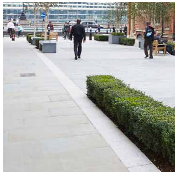
Large flag paving to primary pedestrian pathways
