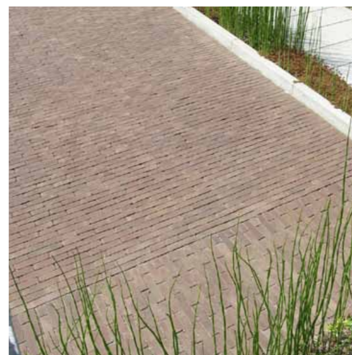
Small unit brick paving to reflect warmth and scale of heritage facades
