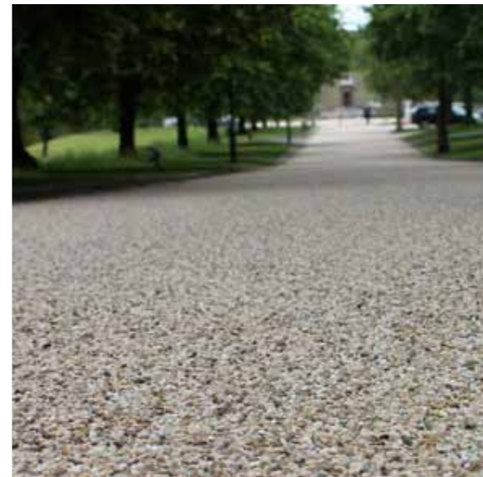
Buff coloured bound gravel to parking courts
