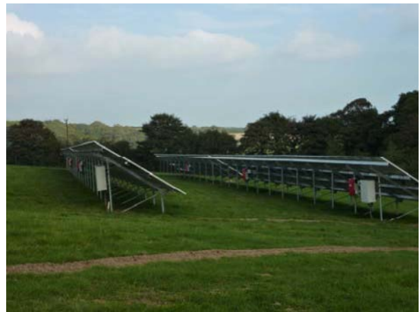
A 49.35kW ground mounted solar PV installation in Cornwall. The installation consists of 116 solar PV panels in 4 rows approximately 65m long
