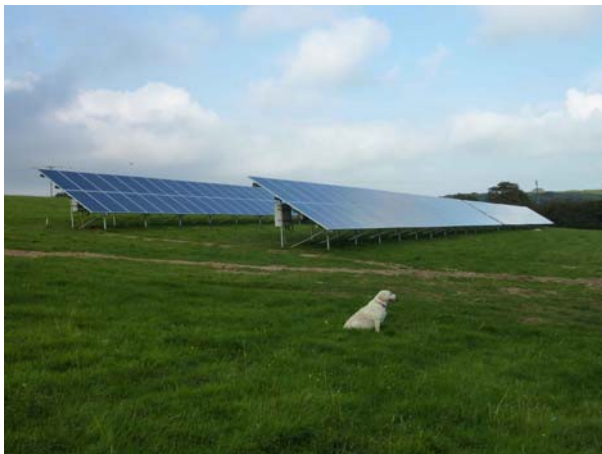
A 49.35kW ground mounted solar PV installation in Cornwall. The installation consists of 116 solar PV panels in 4 rows approximately 65m long
