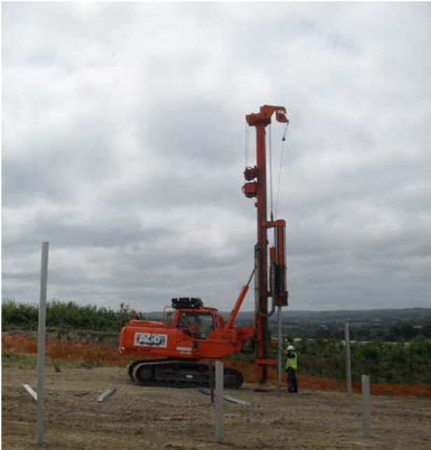
Where there are areas of archaeological interest, and therefore a need to avoid ground disturbance, the use of pre-cast concrete anchors should be considered, as shown here at the 5MW Trefullock solar farm in Cornwall.
