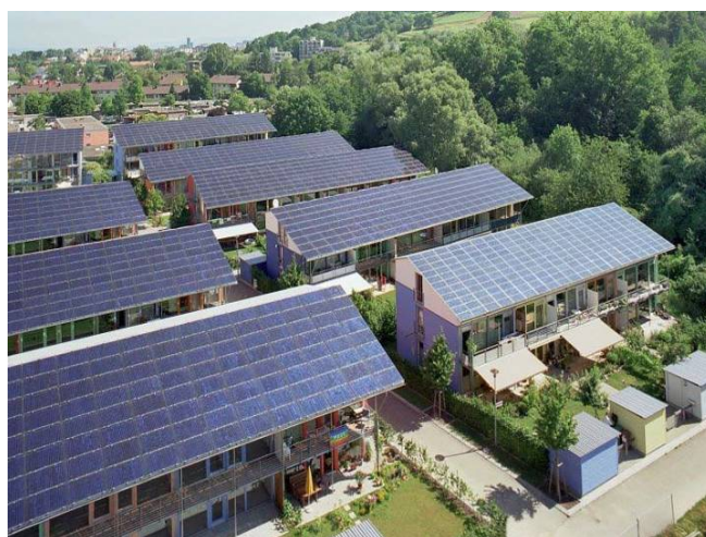
Frieburg, south Germany. The design and orientation of these buildings has been undertaken in order to optimise the potential for installing solar PV. Solar PV levels in Cornwall are similar to solar irradiation levels found in Germany
