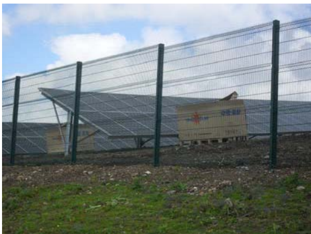
Close welded mesh panel fencing, as shown here at the Wheal Jane solar farm, generally has a low landscape/visual impact while also being versatile and providing a good level of site security.
