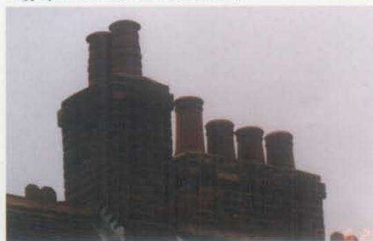
Chimney construction (Guideline 2)
