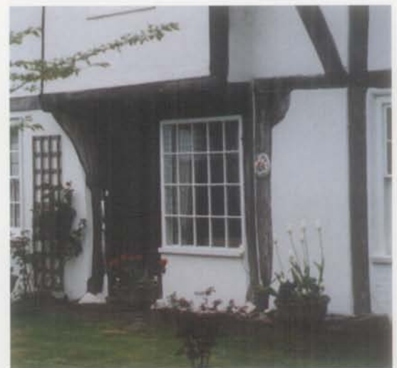
Medieval timber frame with windows of later date (Guideline 1, 6)
