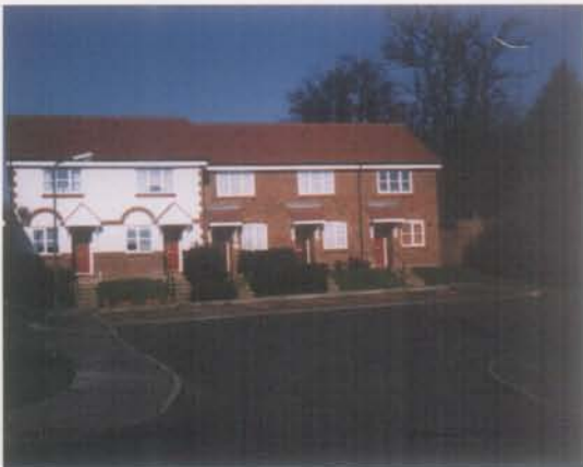
Parking area at Bankside (Guideline 9)
