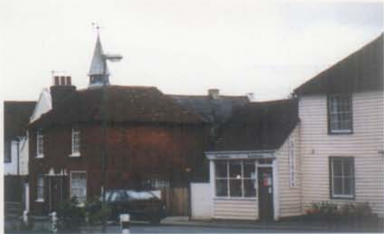
A mix of building styles in The Street (Guideline 1, 2, 3)
