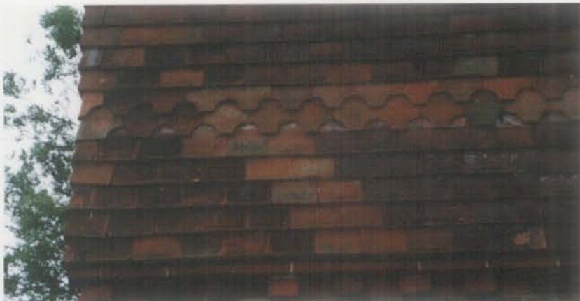
Feature tile hanging using traditional kent pegs (Guideline 1, 3)
