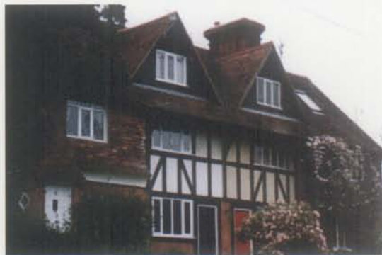
20th c. Half timber and render interpretation (Guideline 1); inappropriate velux window (Guideline 6)
