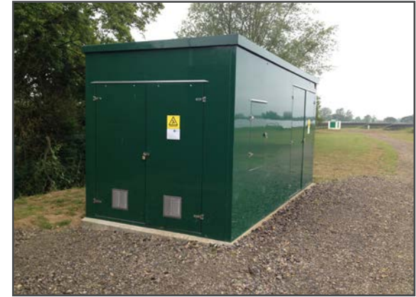
Plate 4 - Typical Substation Cabinet
