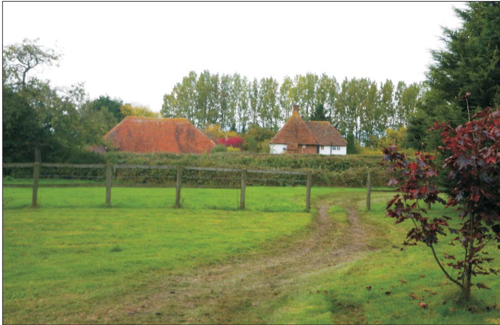
Plate 19: Example of distinctive red peg tile roofs nestled between mature hedgerows. View towards Netters Farm from the grounds of Chilmington Cottage, looking west.
