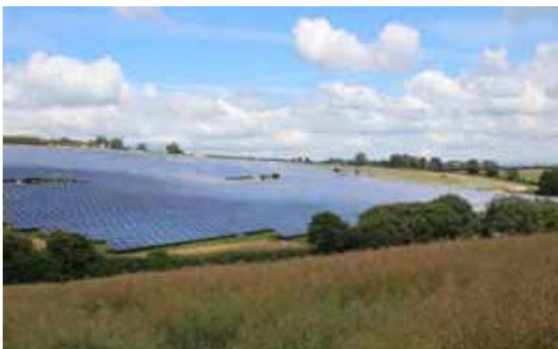
Howton 5MW solar PV farm, Cornwall. Image courtesy of LowCarbon Solar Partners.
