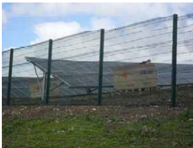
Close welded mesh panel fencing, as shown here at the Wheal Jane solar farm, generally has a low landscape/visual impact while also being versatile and providing a good level of site security
