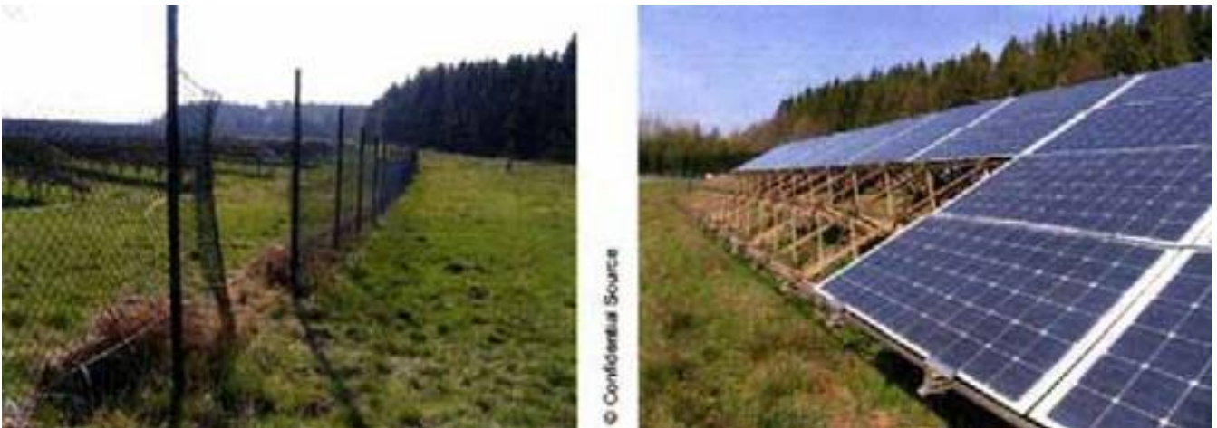
Close welded mesh panel fencing, as shown here at the Wheal Jane solar farm, generally has a low landscape/visual impact while also being versatile and providing a good level of site security
