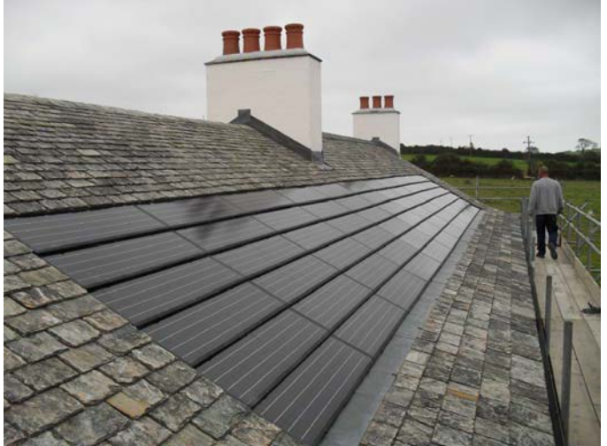
A roof mounted 4kW solar PV installation being installed while the roof is being re-slatted
