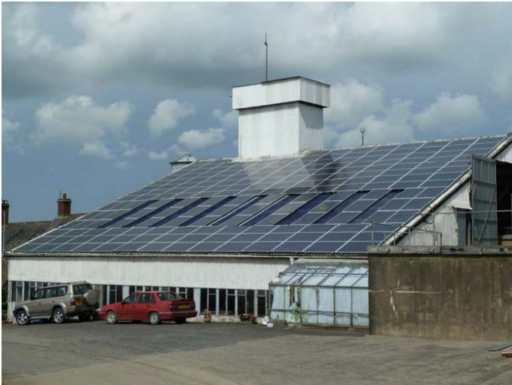
The roof of this agricultural grain drying unit has been clad with solar PV panels which generate a high proportion of the electricity required by the facility. Image courtesy of Clean Earth Energy
