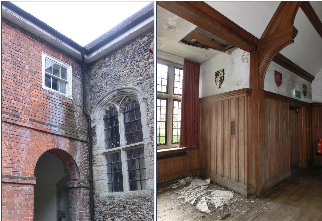
Fig 37 (left). Blocked or broken rainwater goods causing masonry decay in the north-east corner of Cloister Quad. Fig 38 (right). Damage caused by water ingress in the Dining Hall
