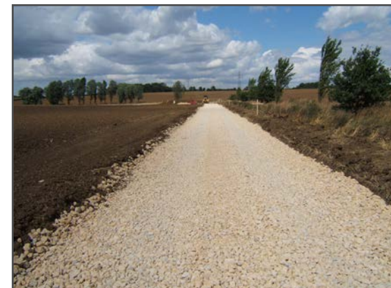
Plate 4 - Typical New Site Access Track
