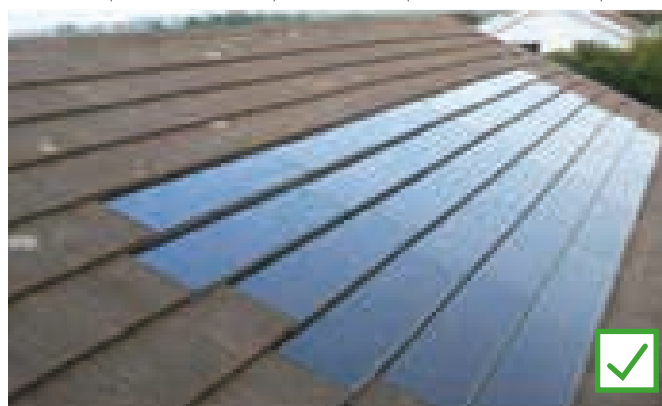
These solar slates are integrated in a tiles roof and are virtually hidden when viewed from the street
