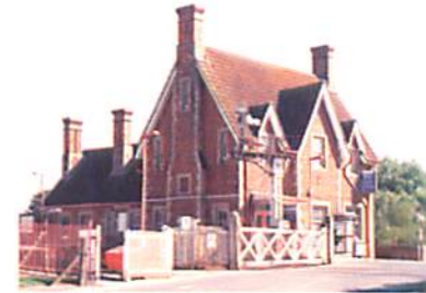
Wye station showing the level crossing
