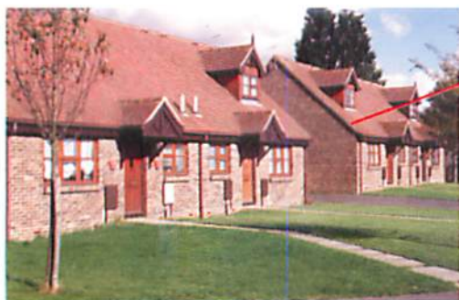
Above: Long's Acre (I) A group of 12 low-cost houses built on the initiative of the Parish Council, in 1992, on part of a field belonging to Miss Hilda Long. This is the only low-cost housing scheme in Wye.
