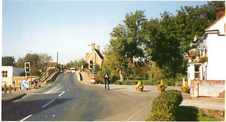
Above: Approach to Wye bridge. In the early 20th century the side walls were removed to accommodate a wider carriageway. More recently, the modern structure was found to be too weak to bear two-way traffic, the carriageway was narrowed and lights installed to control one-way movement.
