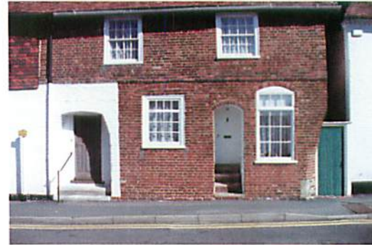
Buildings predominate over landscape in village core (Bridge Street).
