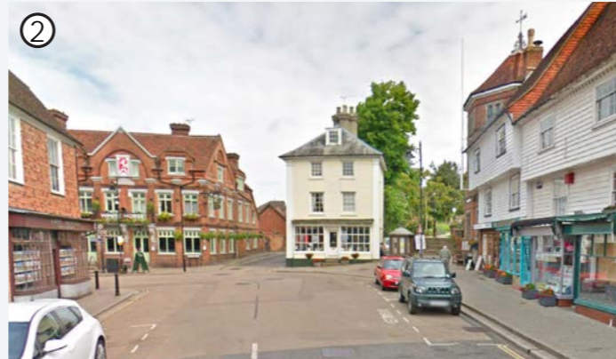
Commercial building terminates a 12m wide secondary street connecting to the High Street. The key building gives a sense of finality and arrival.
