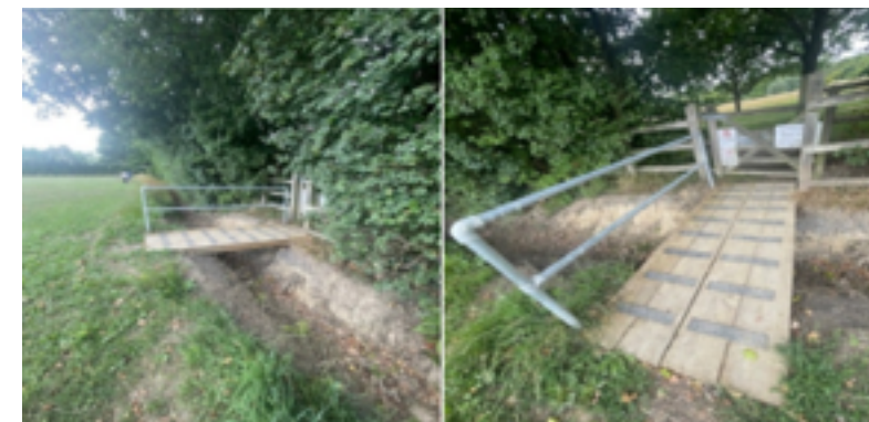
Figure 13. New culvert on a drainage ditch was implemented and a new pedestrian bridge at the Millennium Field, Biddenden.
