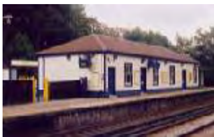
Pluckley Station (built 1842)
